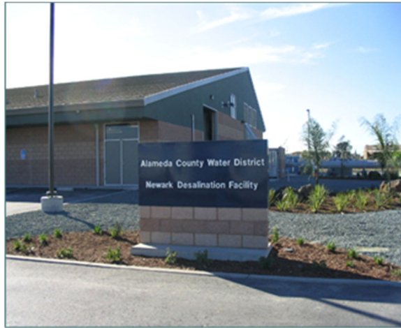
Figure 5-1 The Newark Desalination Facility
