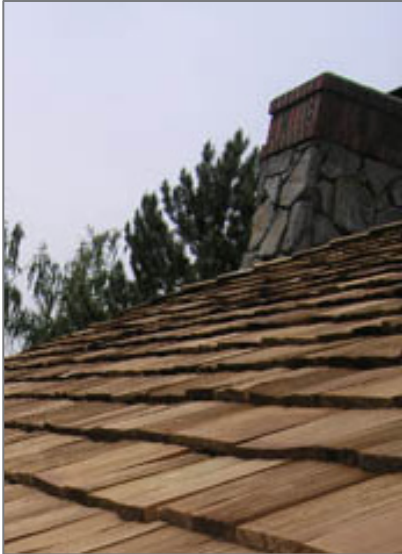
Wood shingle roof Courtesy of Gutter Glove
