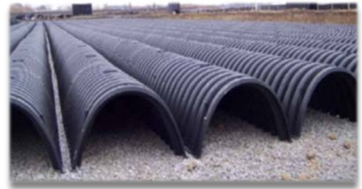
Figure 2-5 Subsurface infiltration system (Source: Conteches.com)
