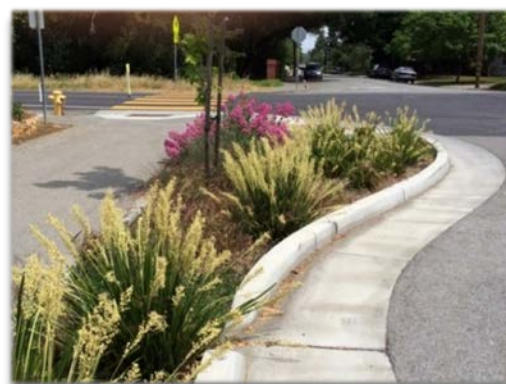
Figure 2-1 Stormwater curb extension, Rosita Park, Los Altos (Source: City of Los Altos)
