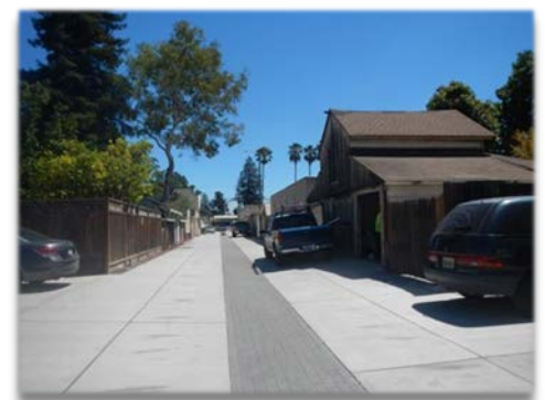
Figure 2-4 Infiltration Trench, San Jose (Source: City of San Jose)
