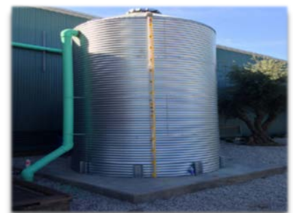
Figure 2-7 Rainwater harvesting cistern, Environmental Innovation Center, San José (Source: City of San Jose)
