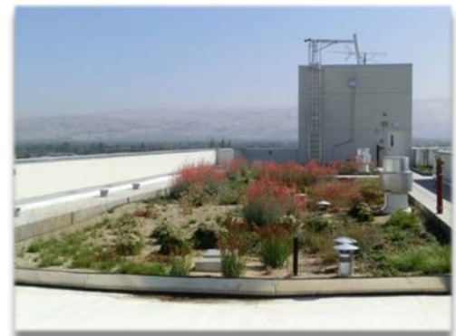
Figure 2-6 Green Roof at Fourth Street Apartments, San José (Source: EOA)
