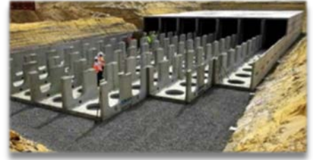
Figure 2-8 Subsurface vault under construction (Source: Conteches.com)
