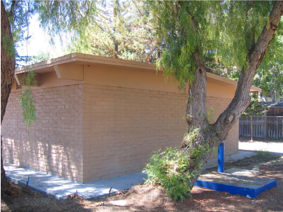
Figure 2-52. Wolfe-Evelyn Pump Station Building
