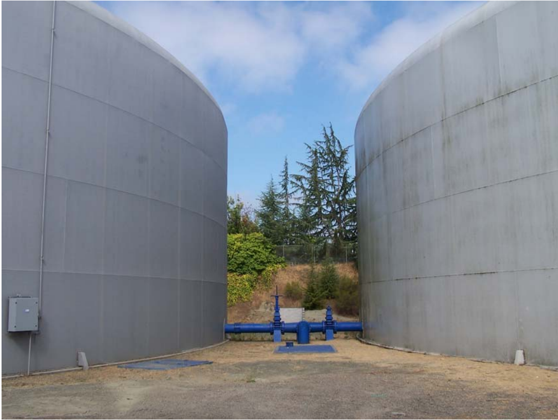
Figure 2-11. Mary Carson Tank 2 (left), Tank 1 (right)
