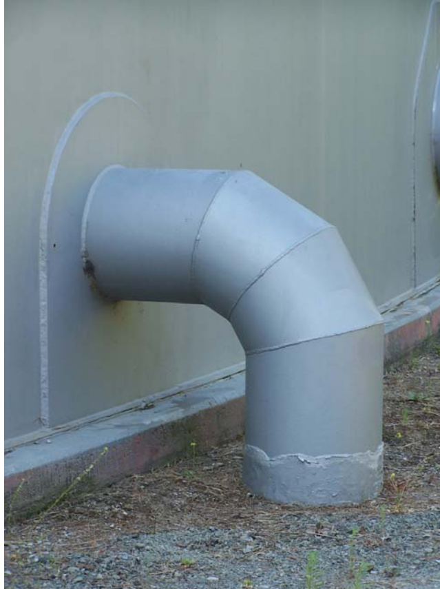
Figure 2-13. Mary Carson Tank 2 Overflow Pipe
