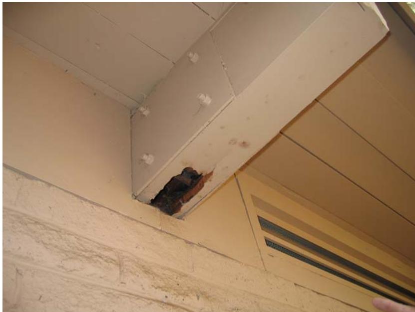
Figure 2-16. Mary Carson Pump Station Building – Repaired Roof Beam
