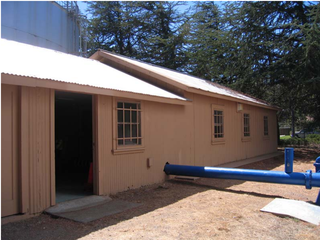
Figure 2-45. Central Pump Station
