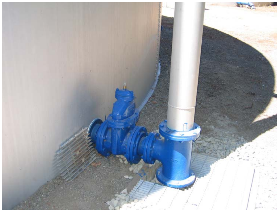
Figure 2-39. Tank #1 Riveted Overflow and Drain to Catch Basin
