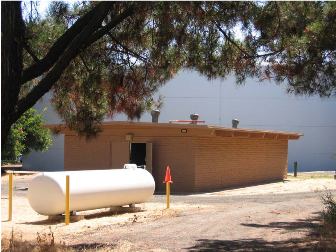
Figure 2-23. Wright Avenue Pump Station Building (Propane Tank in foreground)
