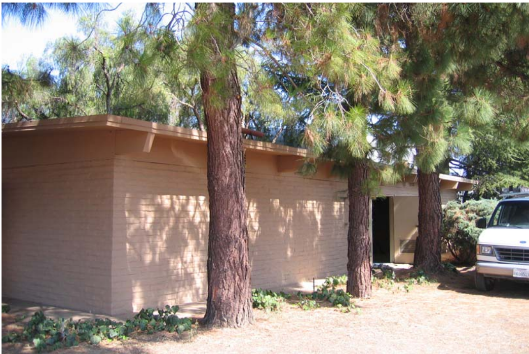
Figure 2-14. Mary Carson Pump Station Building
