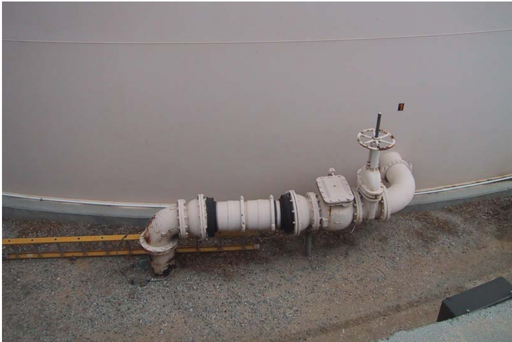
Figure 6-3. Flexextend Hardware (EBAA) Installed for side Entry Pipe (Example)
