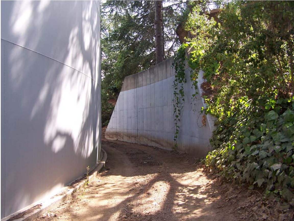
Figure 2-15a. Retaining Wall (right), Tank 2 (left)
