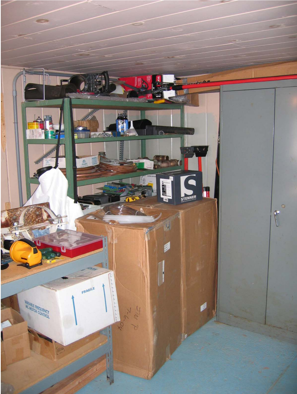
Figure 2-47. Central Pump Station Storage Shelves
