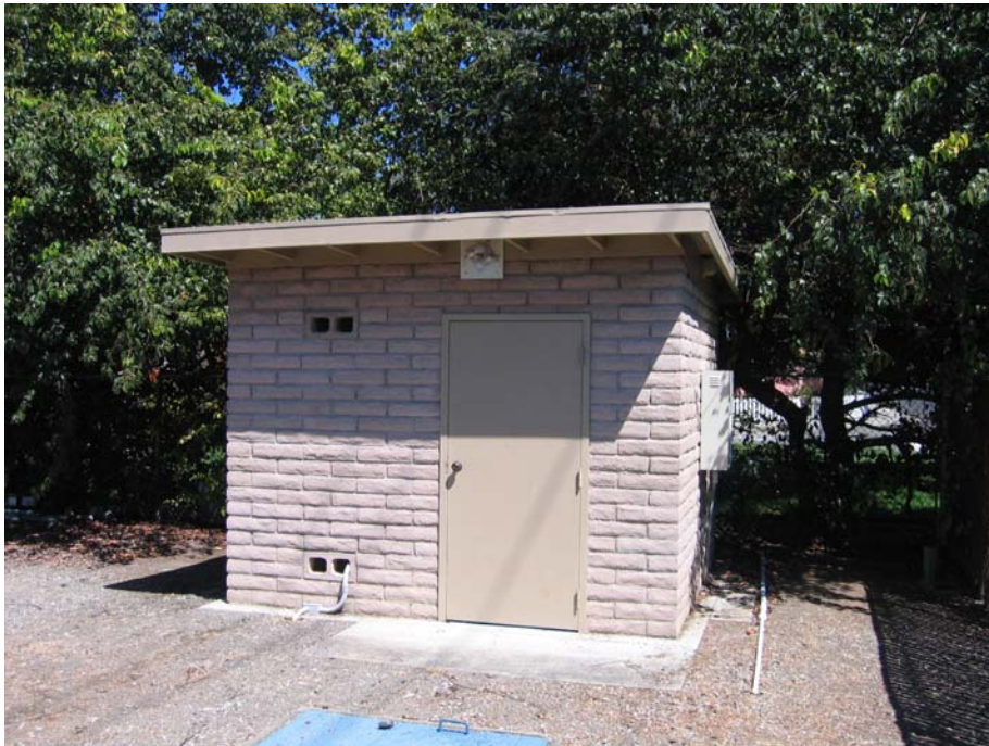
Figure 2-67. Schroeder Well – Control Building
