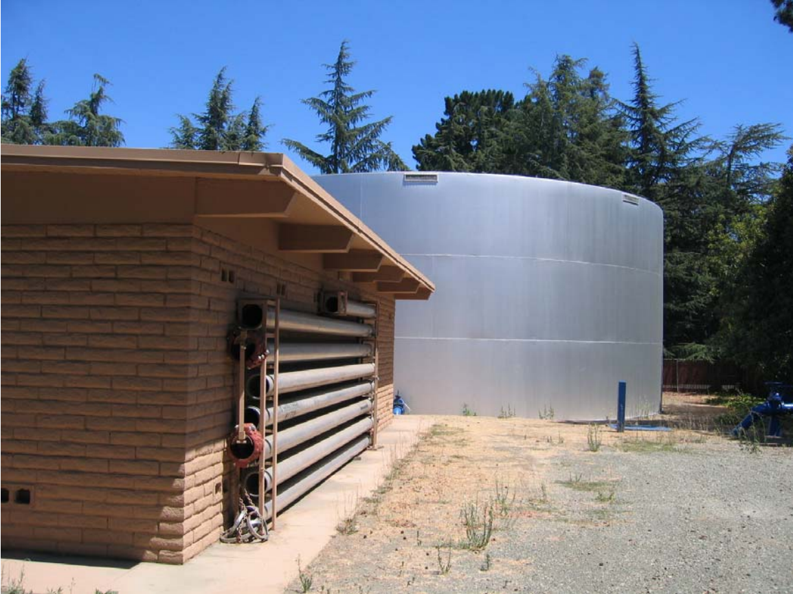
Figure 2-34. Hamilton Tank #3 (background) and Pump Station Building
