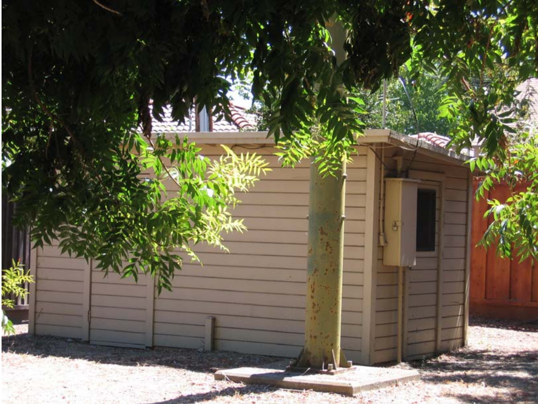
Figure 2-65. Losse Well – Control Building
