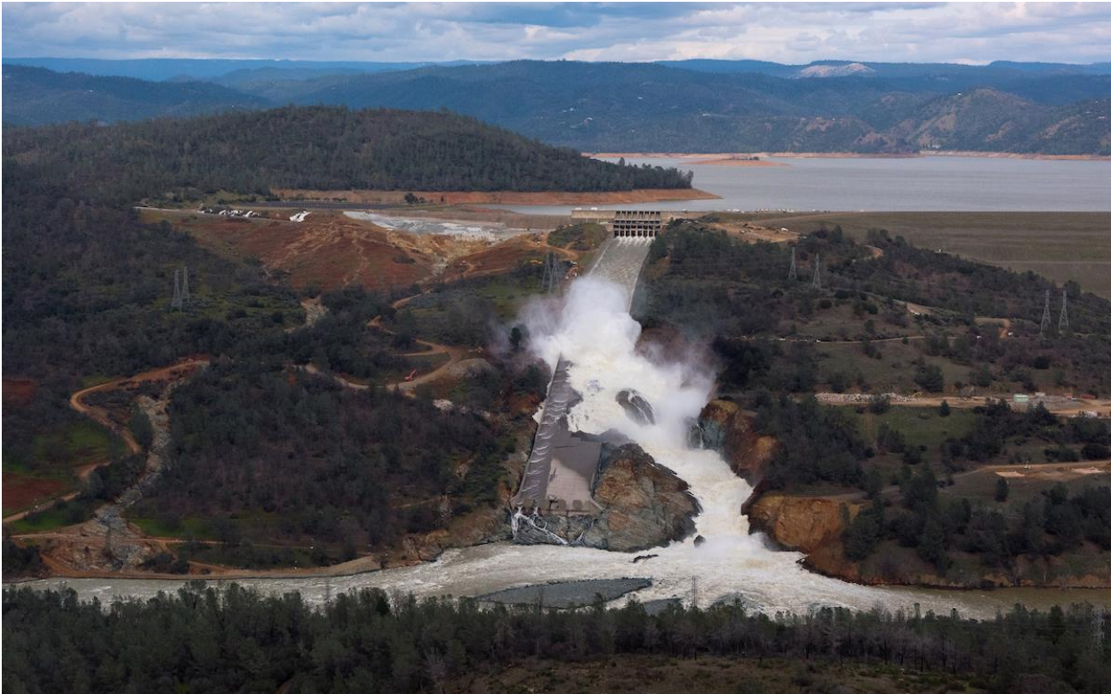
An aerial view of the damaged Oroville Dam spillway on February 26, 2017
