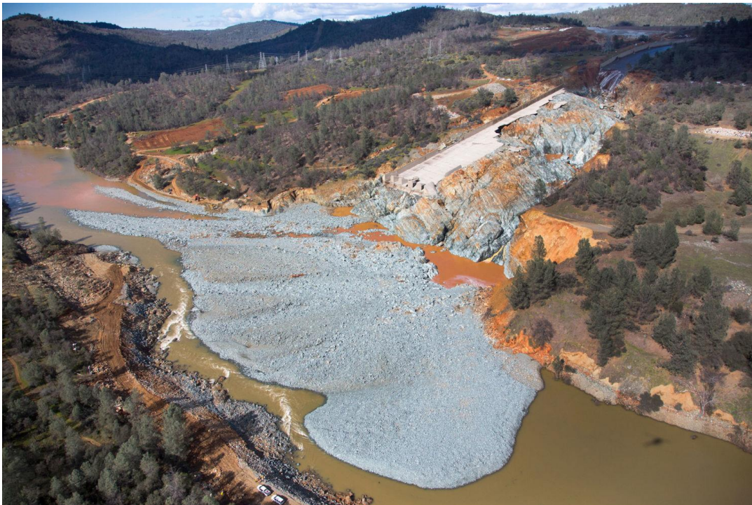
An aerial view of the damaged Oroville Dam spillway in California, and the debris field just below, in February 2017. California Department of Water Resources
