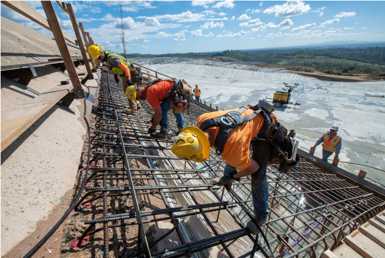
Workers repair the damaged Oroville Dam spillway in Northern California in March. California Department of Water Resources
