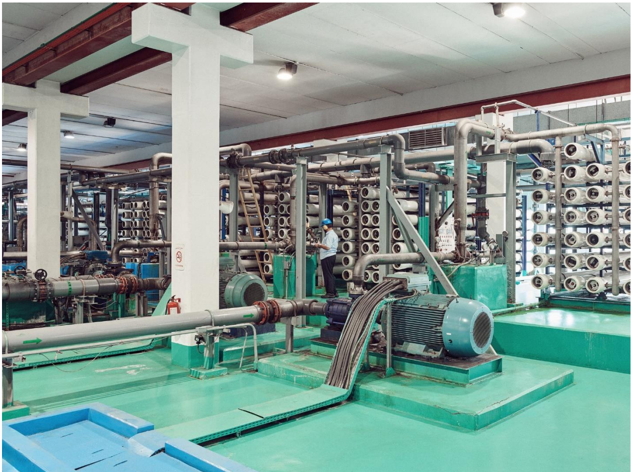
Electric water pressure pumps and reverse-osmosis membrane tubes at the Sawaco Desalination Plant in Jeddah, Saudi Arabia.
