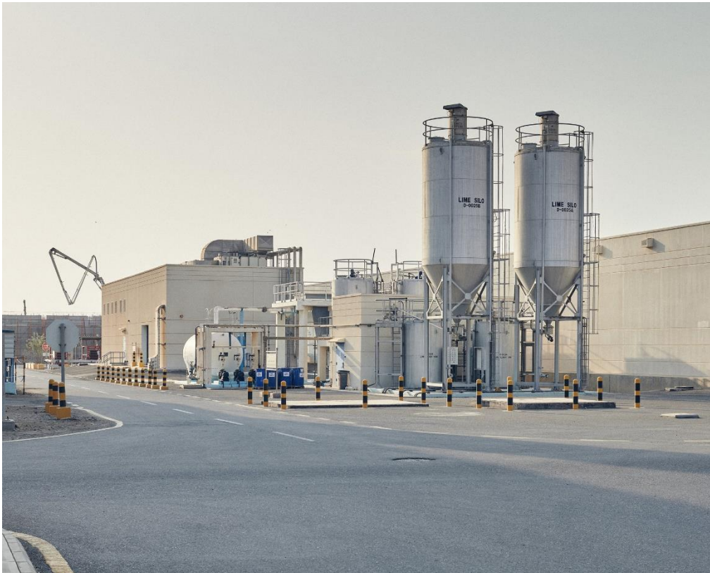
Lime silos outside the Kaust facility holding chemicals used to treat the water after it is desalinated.
