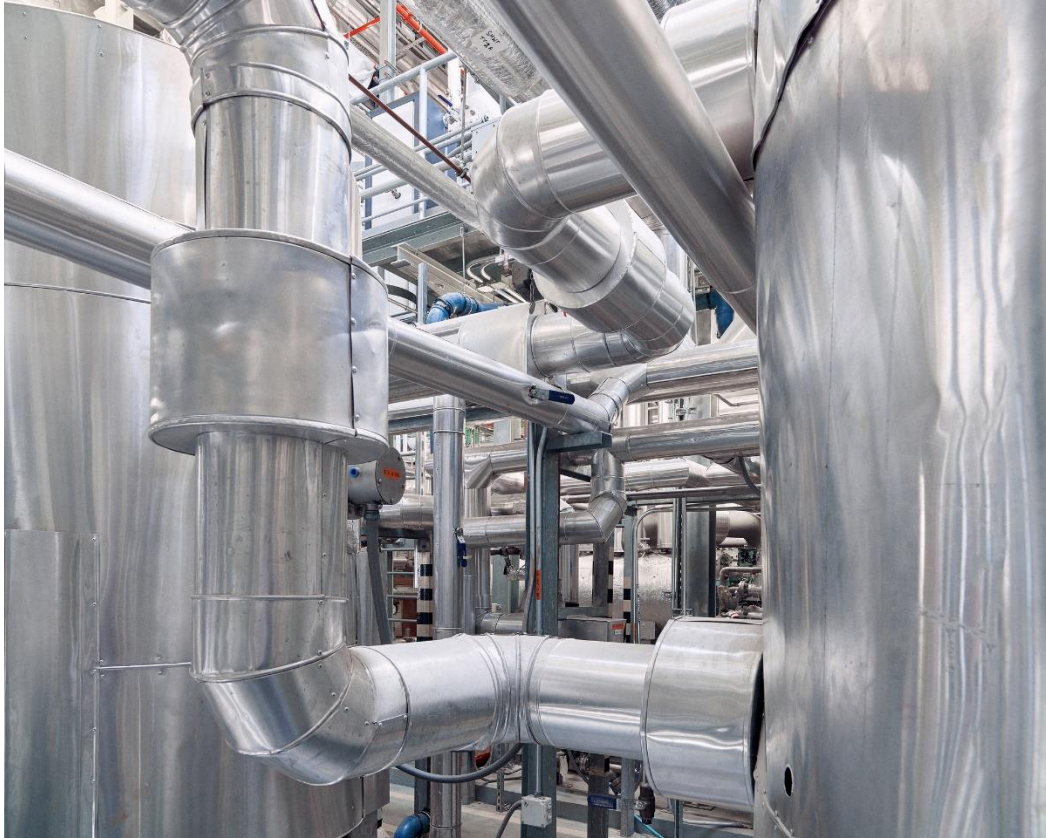
A solar-powered pilot desalination project facility at Kaust.
