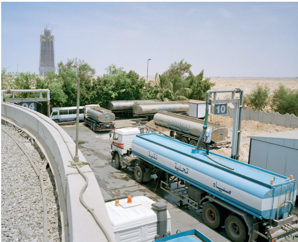
There are no water distribution pipes in this part of Jeddah, so the desalinated water is distributed by truck.
