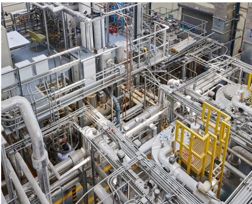
The small pilot plant, which uses solar energy to heat the water for desalination.
