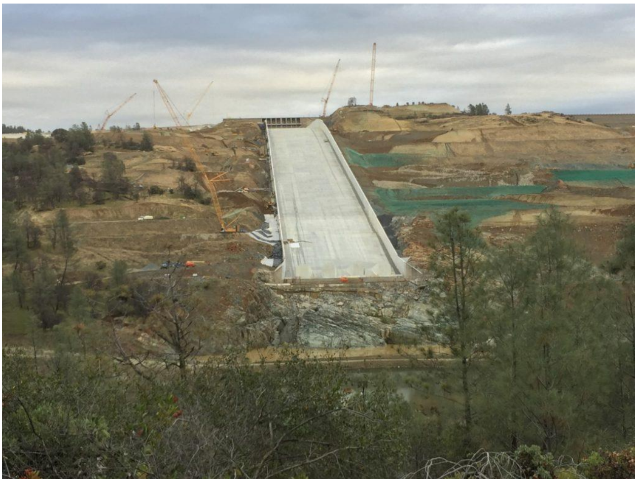
Oroville Dam Spillway Reconstruction (Joel Pollak / Breitbart News)
