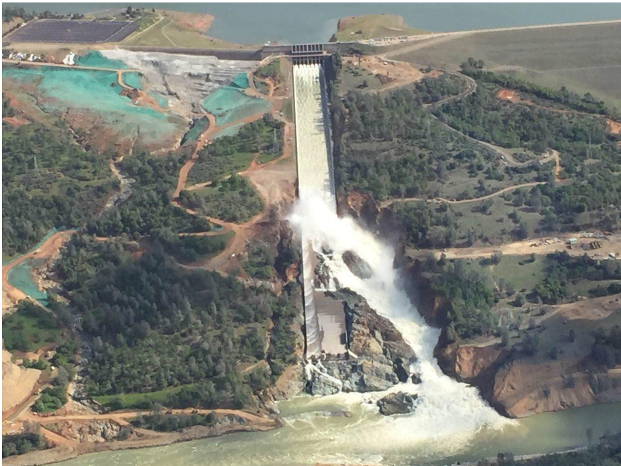
Oroville Dam Spillway (Joel Pollak / Breitbart News)
