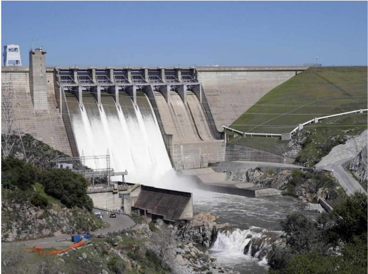
Water flows from five of the eight flood gates at Folsom Dam Friday, March 18, 2016, in Folsom, Calif. Rich Pedroncelli / AP Photo
