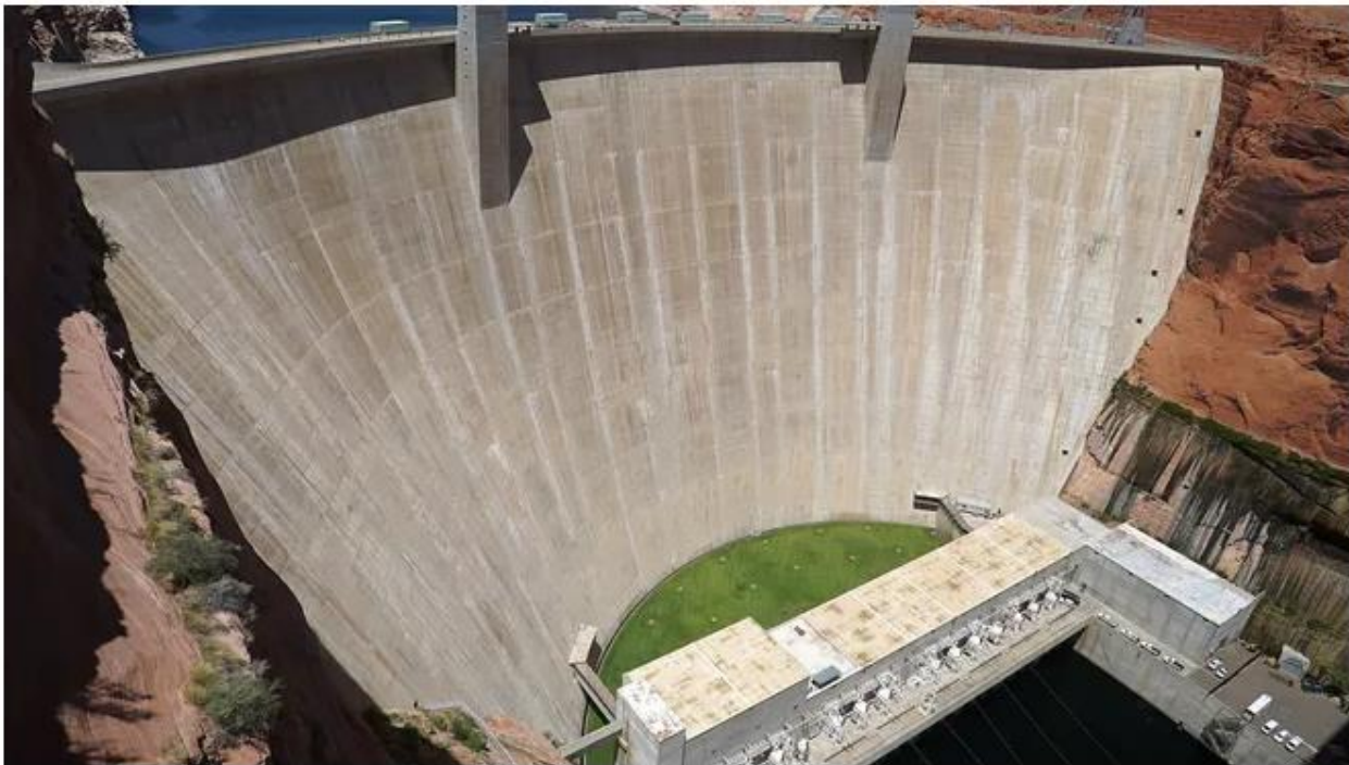
The Glen Canyon Dam, which impounds the Colorado River to create Lake Powell, was originally designed to be 16 feet higher, making it the same height at the Hoover Dam on Lake Meade in Nevada. Engineers shortened the dam, lowering the reservoir's height, to protect Rainbow Bridge, North America's largest natural rock bridge, which is about 50 miles north of the dam. Trevor Hughes, USA TODAY
