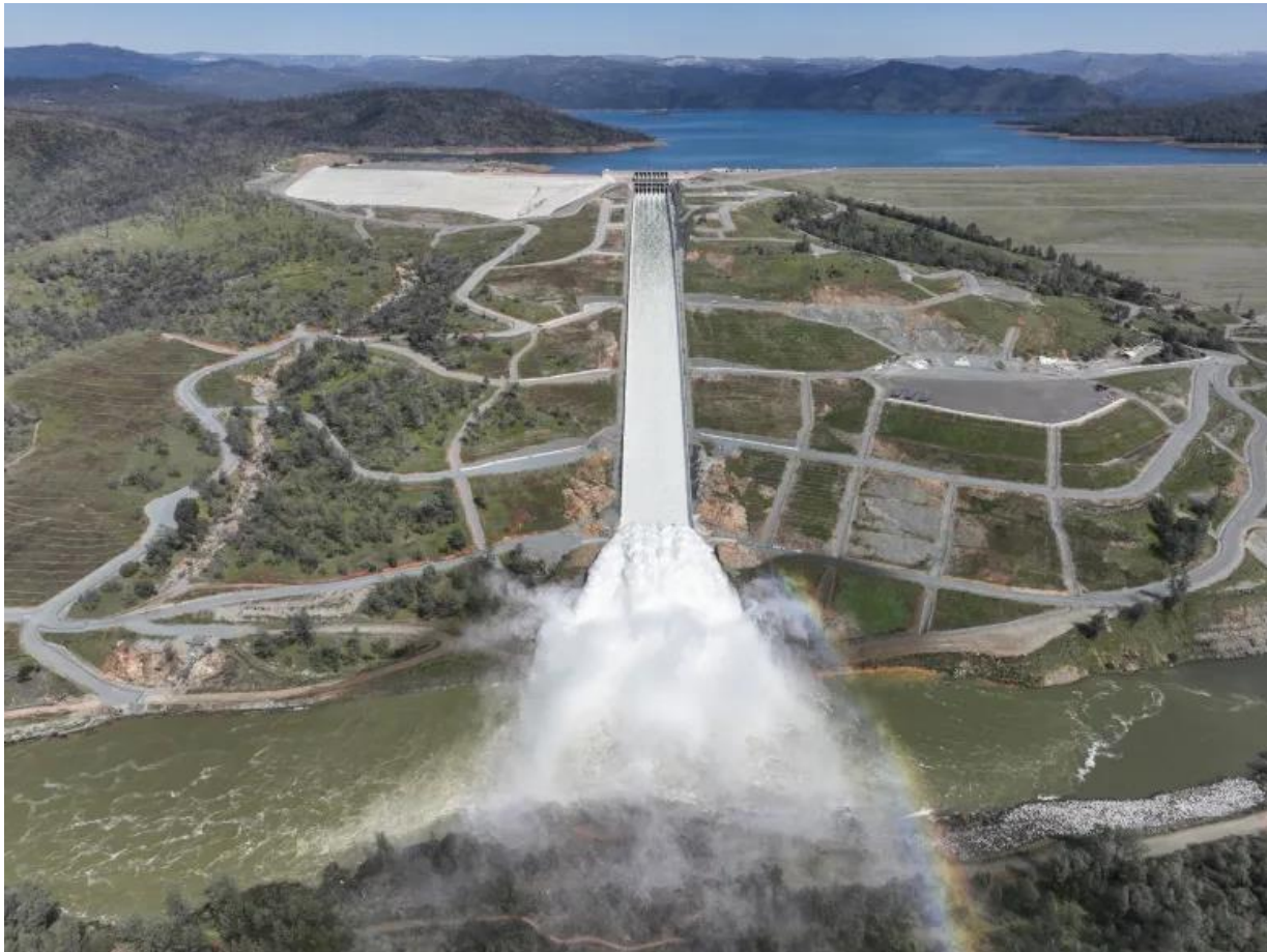
A drone provides an aerial view of a cloud mist formed as water flows over the four energy dissipator blocks at the end of the Lake Oroville Main Spillway. (Ken James / California Department of Water Resources)
