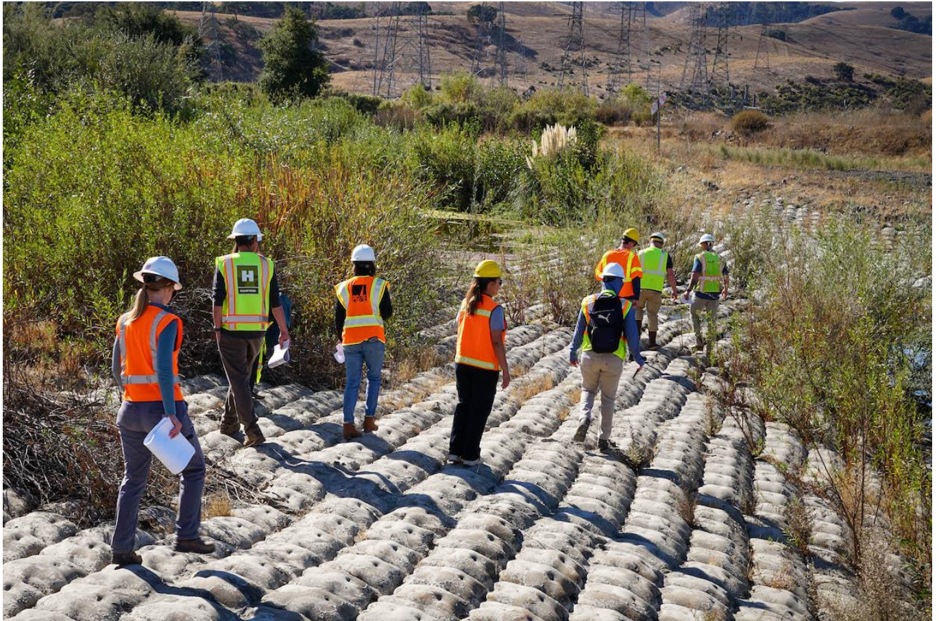
Officials inspect the PG&E gas pipeline protective apron over Alameda Creek near Sunol. Photo by California Trout
