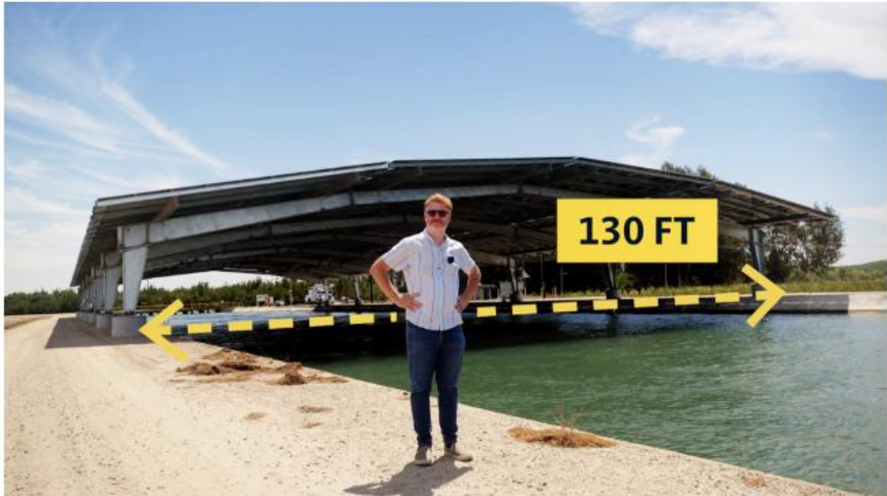
Project Nexus is also testing out a wider, 130-ft span. Credit: Fig. 1 by University of California
