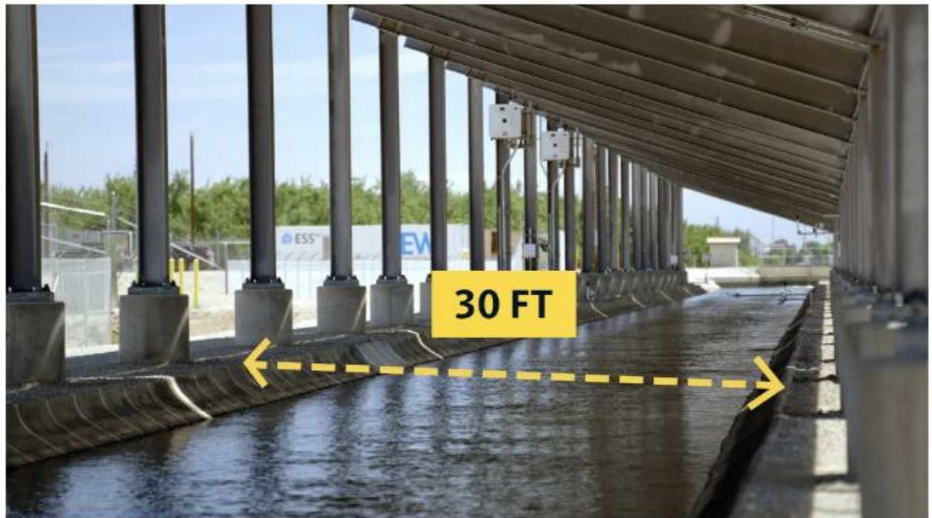
Project Nexus is testing out a 30-ft span of solar panels over one stretch of canal. Credit: Fig. 1 by University of California
