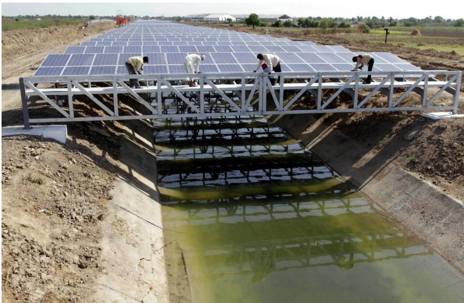
Construction of an earlier project above a canal near Ahmedabad, India, in 2012. Credit...Ajit Solanki/Associated Press
