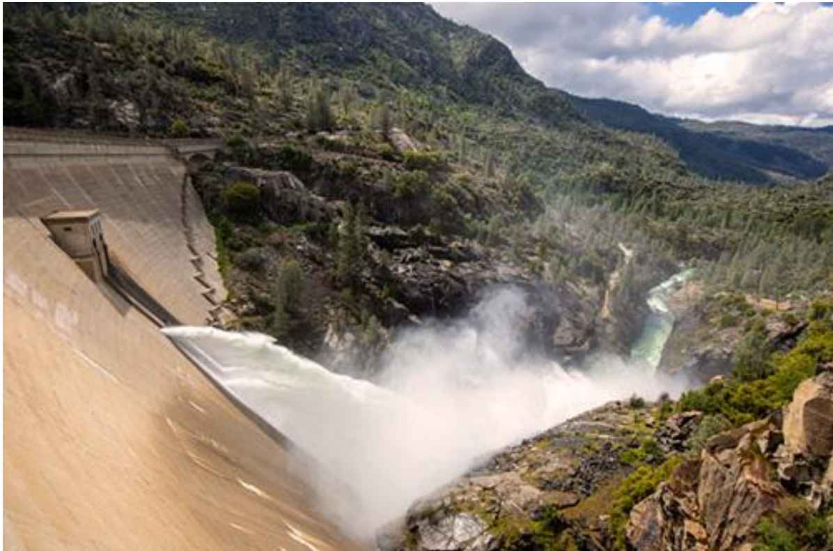
The Michael M. O'Shaughnessy Dam, part of the Hetch Hetchy Water System. Photo credit: SFPUC
