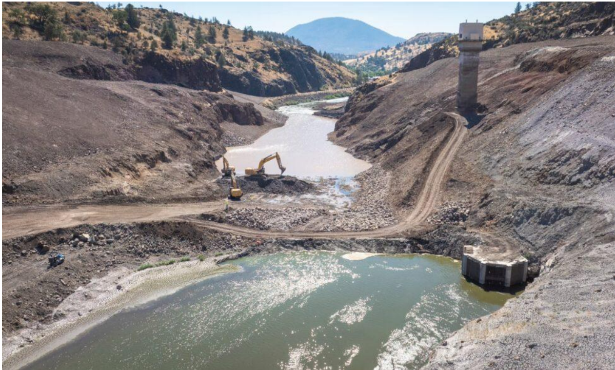
Klamath Dam removed, Photo credit Swift Films
