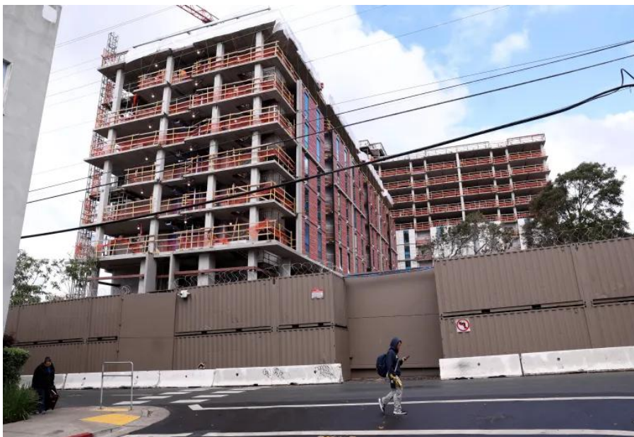
Work continues on UC Berkeley's People's Park Housing Project in Berkeley, Calif., on Tuesday, Oct. 14, 2025. Neighbors in Berkeley delayed construction of a new UC dormitory there for three years, claiming the students would create noise pollution. (Jane Tyska/Bay Area News Group)
