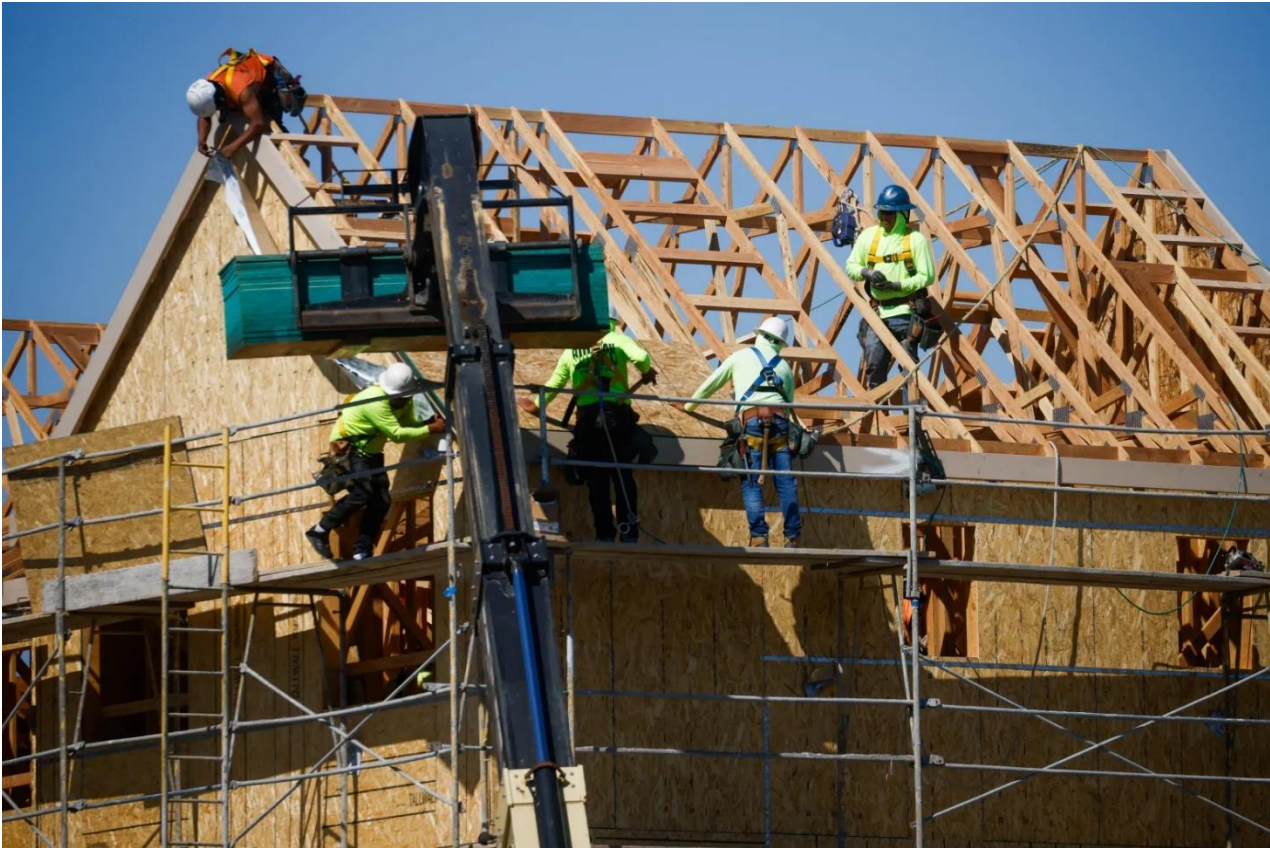
Construction workers build housing across the street from Campbell Park in Campbell, Calif., on Tuesday, June 16, 2026. (Shae Hammond/Bay Area News Group)
