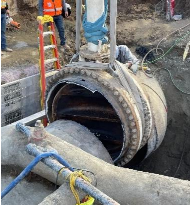
Valve V-442 Removal
