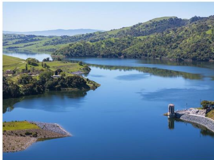
Calaveras Reservoir - 2024. Photo courtesy of San Francisco Public Utilities Commission.
