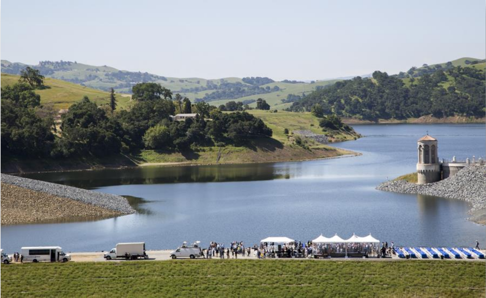
New Calaveras Dam – May 2019
