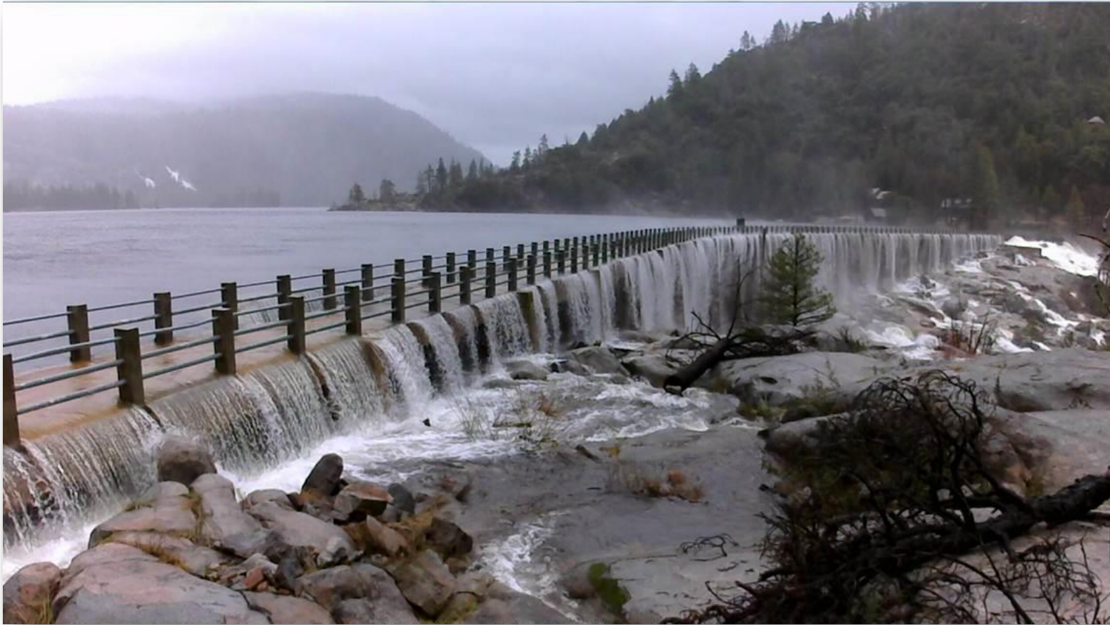
Lake Eleanor Overtopping/SFPUC, January 2017
